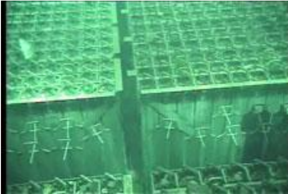
Fig. IV-5-12 Condition of the spent fuel pool (Unit 4)
