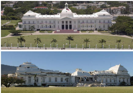
Fig.2. National Palace before and after.
